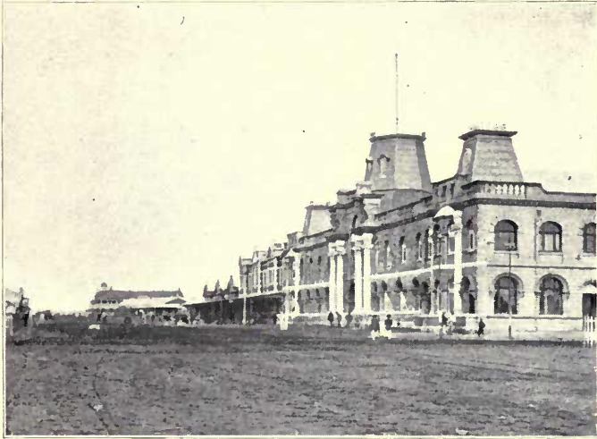
AGENCY BUILDINGS AND NEW HIGH COURT, BULUWAYO.
